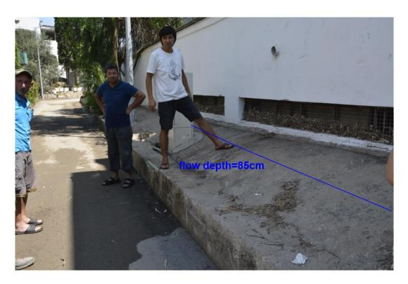
Figure 4.4: Observer showing the flow depth by his foot (37.031412N 27.406703E)
