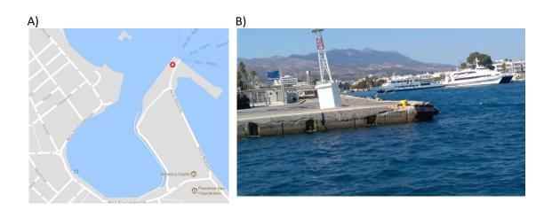
Figure 7.34: Failure on the ground of the lighthouse were occurred by the strong shaking of the earthquake and structural problems of the dock. A) Location of the light house B) Port structure deformation due to the earthquake
