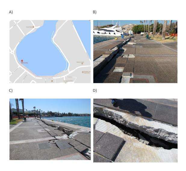
Figure 7.33: A) Damage line at the dock of port B) Damage at the dock of port C) Damage at the dock of port D) Distancing of the materials of the dock
