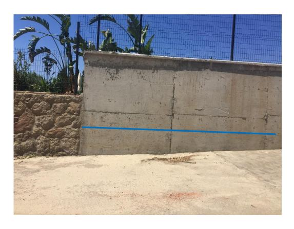
Figure 4.13: Wave trace on the sidewalls of the road, Karaincir Bay (27.300718E 36.973574N)
