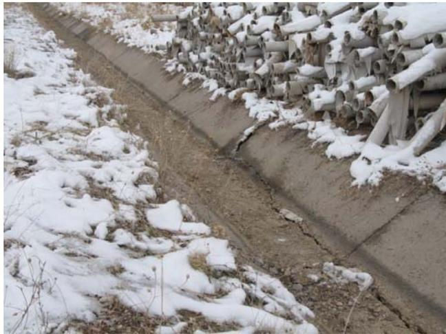
Figure 7.4: Deformation on the irrigation canal depends on the compression regim
