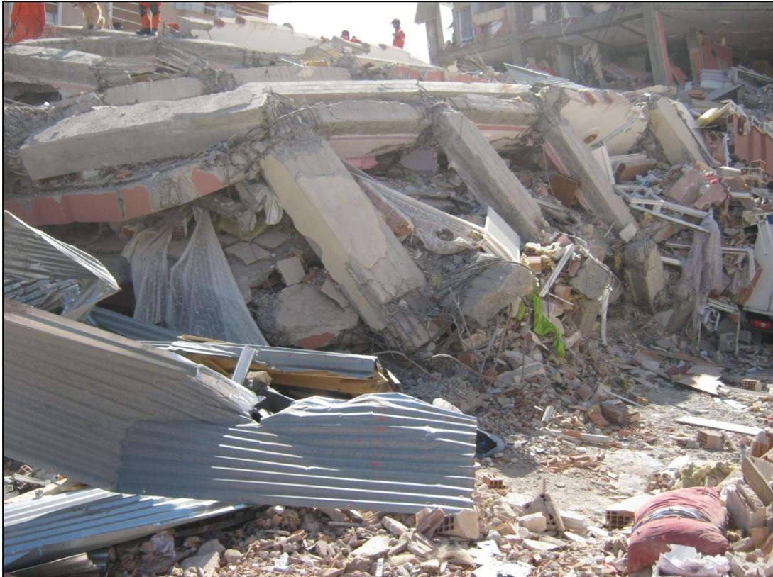
Figure 17.3: Crumbly concrete example
