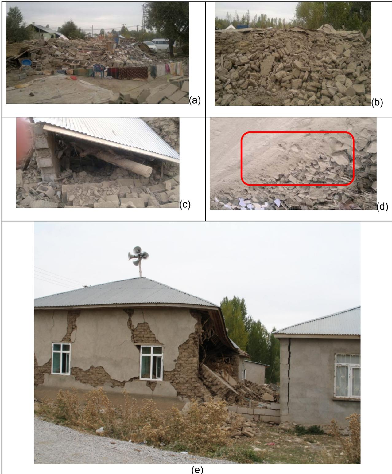
Figure 17.6: a) Briquet filled collapsed building, b) Adobe filled collapsed building
