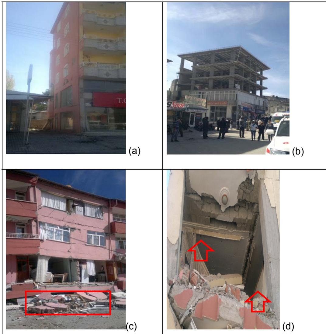
Figure 17.1: Examples of weak storey and slab effect. (a. Weak storey, b. Weak storey and asmlen slab, c. Ground floor destroyed. d. Heavy slab)
