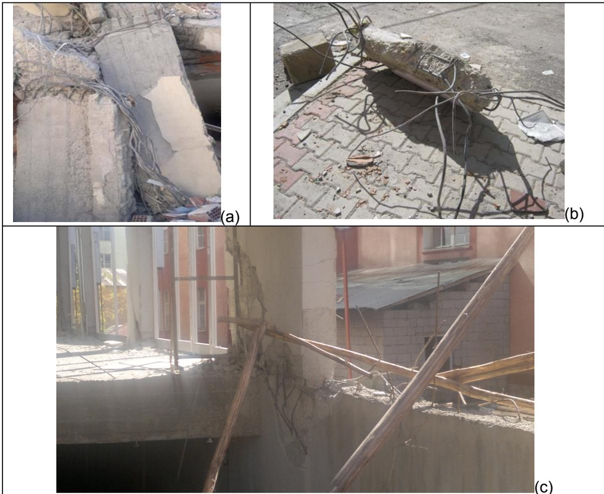
Figure 17.5: a) Striped reinforcement , b) Striped reinforcement
